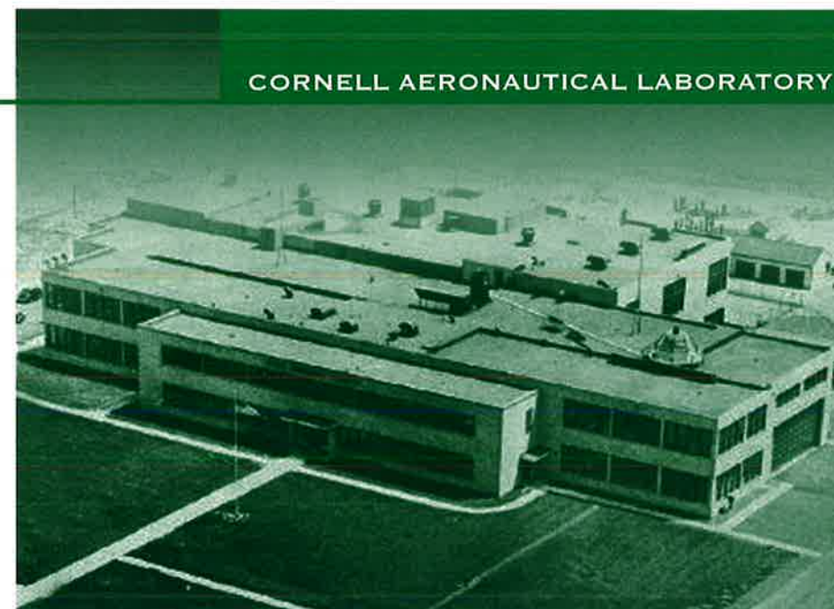
The principal building of the Research Laboratory.
